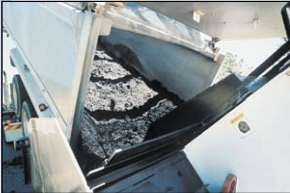
Even this mix can make a good pavement if it is run through a Roadtec MTV.
